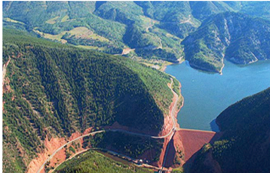
Seventeen Western Colorado entities came together in 2013 to cooperatively retire the debt to the federal government for construction of Ruedi Reservoir. The collaboration will benefit a diverse group of water users for environmental, economic, agricultural, municipal and recreational use in Western Colorado.
